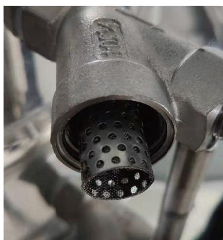
Remove perforated filter to clean
